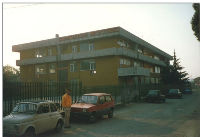
Building before Milestone's foundation.
